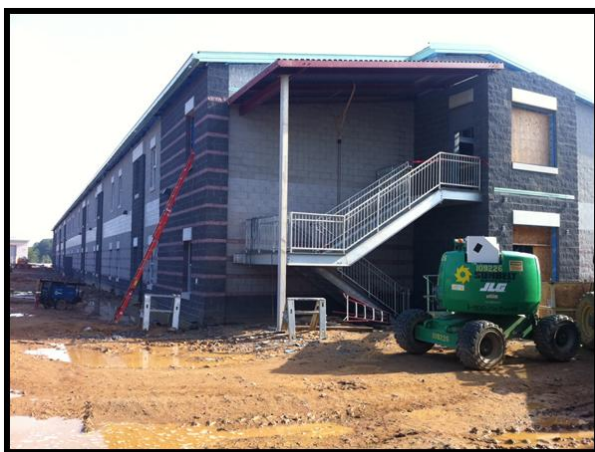
Figure 11: Masonry Veneer – Taken by Kendall Mahan
