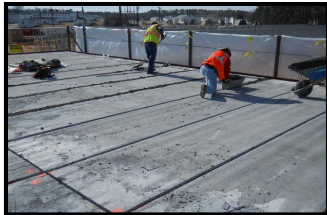
Figure 5: Grouting – Courtesy of Barton Malow
