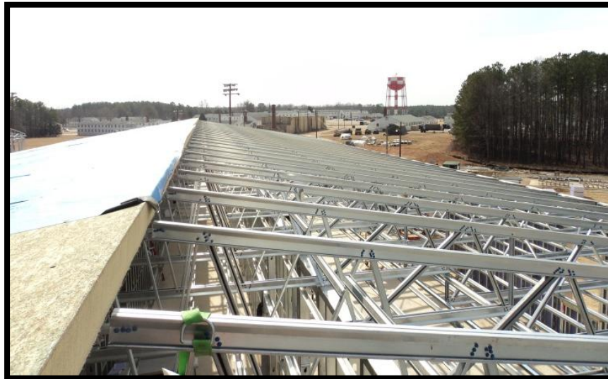
Figure 14: SIPS Erection – Courtesy of Barton Malow
