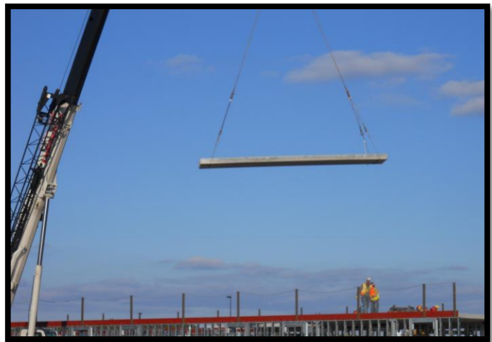
Figure 2: Setting Hollow-core Planks – Courtesy of Barton Malow
