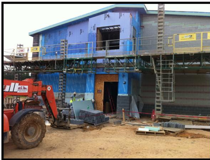
Figure 8: Scaffolding – Taken by Kendall Mahan
